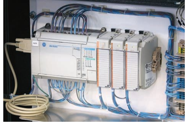
Figure 1-29 Single-ended PLC application.
